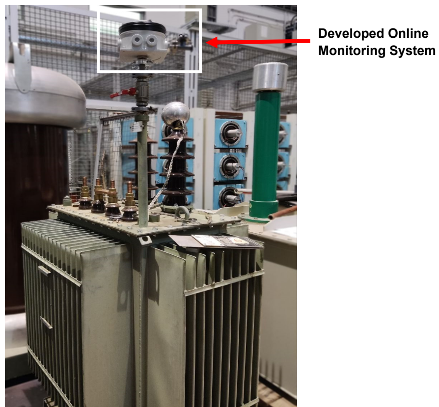
Figure 2: Overview of the hermetic transformer with the installed online monitoring system
